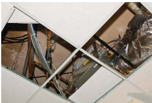
Cramped work area above ceiling—new VAV, control valve and actuator
