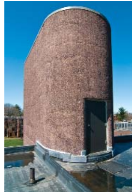
Rooftop Mechanical Access
