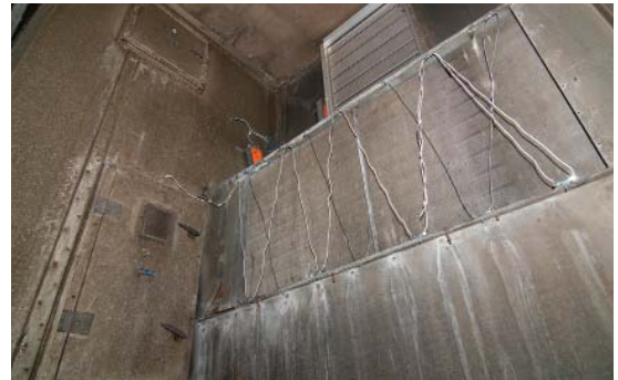
Typical installation of new damper and actuators with tight access
